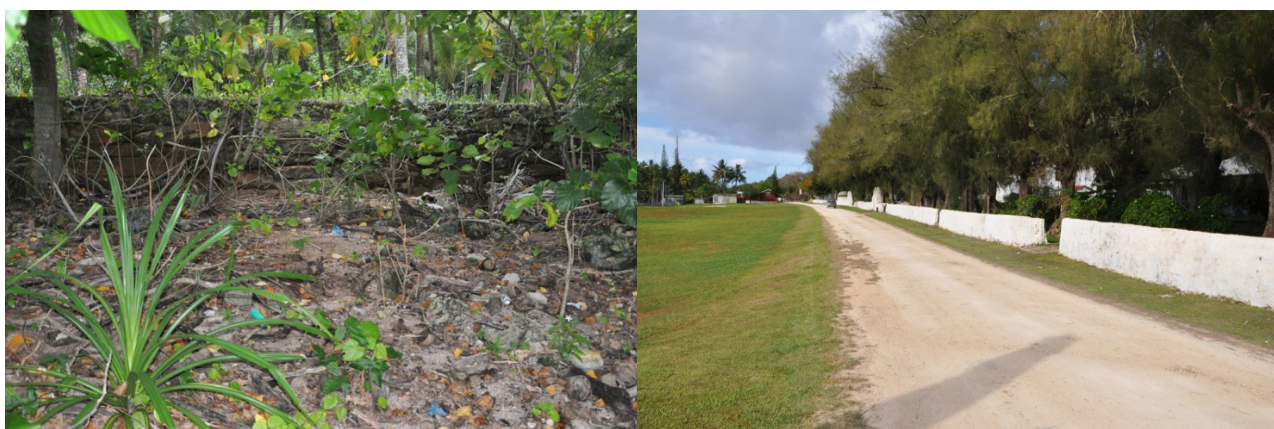
Figure 35. Examples of more appropriate 'seawall' structures for the Oneroa frontage. Left: The wall is located close to the level of the road and will provide much more protection to the road than a similar sized structure located at or close to the shoreline. Right: the wall around the church – even if wave run-up reaches the wall, the wall will prevent water entering the churchyard if the openings are blocked up.
