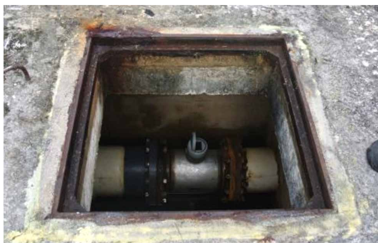
Figure 9. A bulk meter installed in a manhole on the pipeline. Photo: Louis Bouchet.
