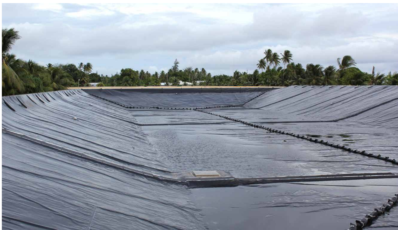
Figure 10. Airport reservoir (storage tank 3), showing the new lining. Photo: Joseph Cain.
