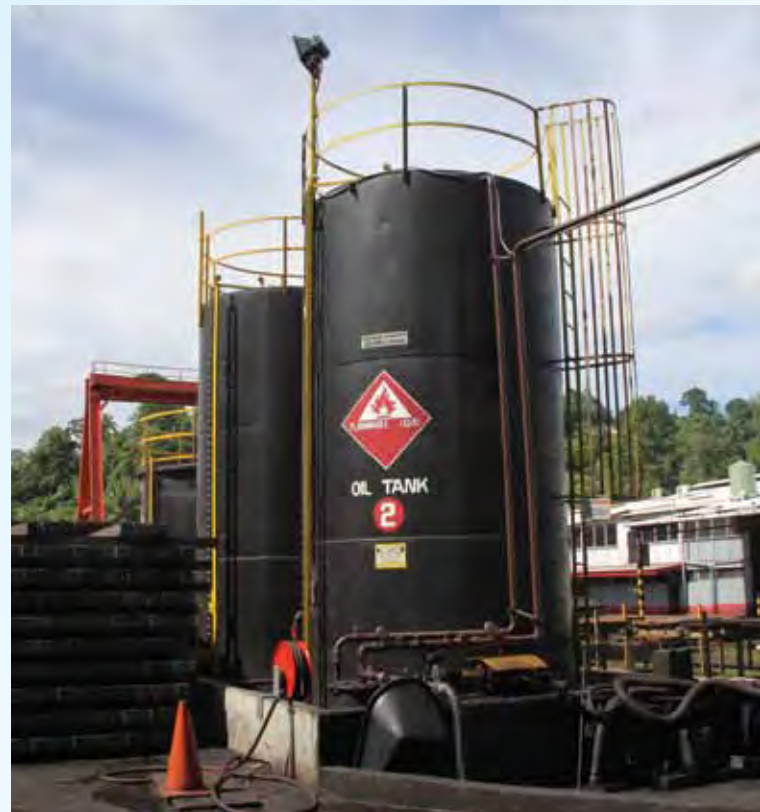
Used oil storage tanks, Fletcher Pacific Steel, Fiji. Photo credit: D. Haynes.
