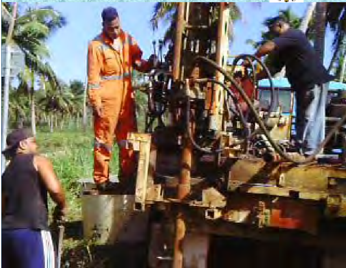
Drilling of 3 monitoring boreholes
