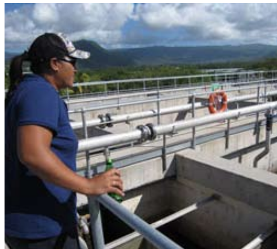
Jammie Saena of the Samoa Water Authority checks one of the tanks that separates solid and liquid waste
