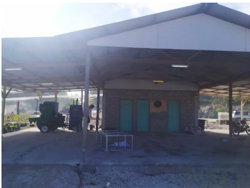
Figure 1: Waste segregation building at the waste facility
