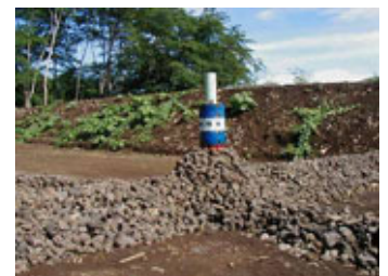
Pic.2 Leachate collection and gas venting pipe
